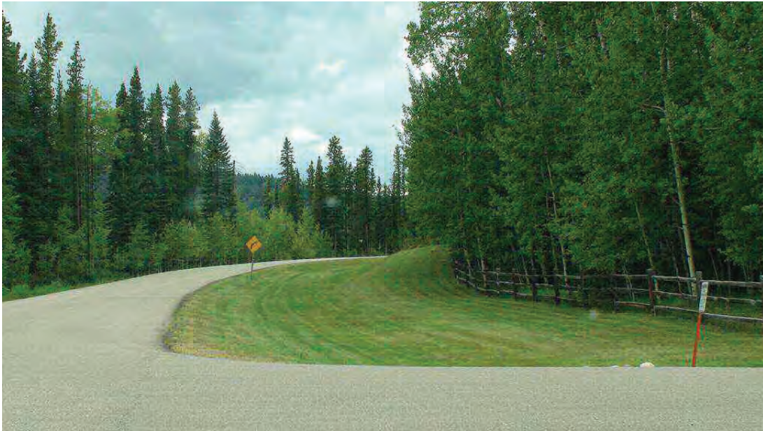
Photo #2-4 Mowed grass swale
