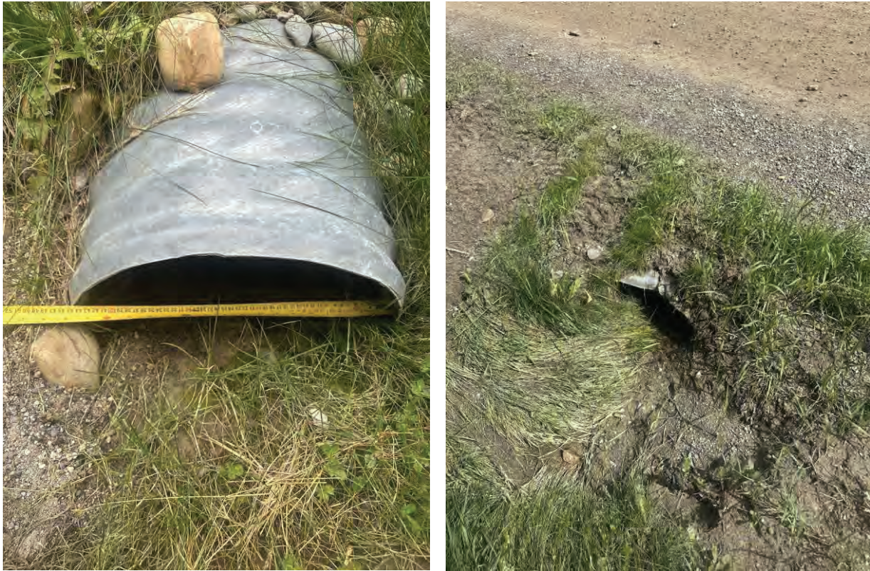
Figure 5.0: Crushed or Damaged Culverts
